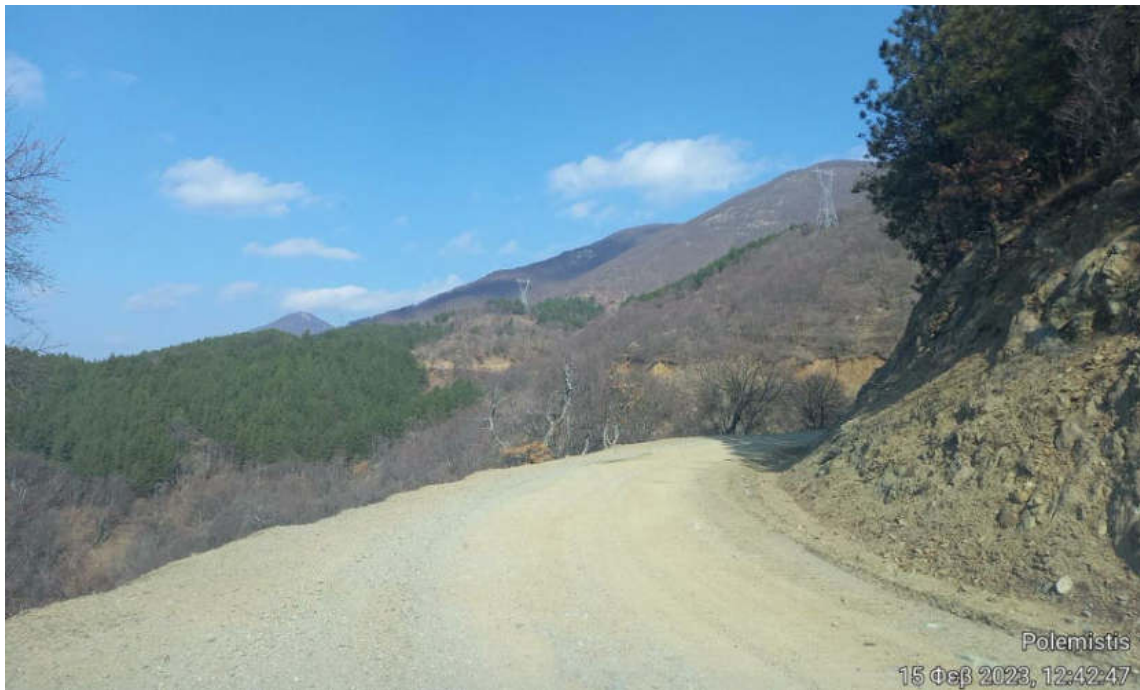
Photo 14-1: Illustration of the area where the MT cable will run underground (1 of 2)
