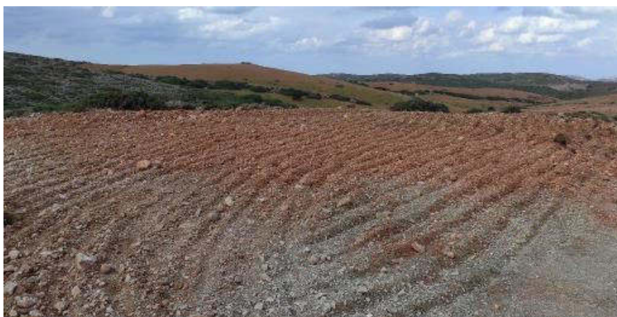
Figure 6.6- 4: Restoration of the A/G square and return to agricultural use (PPC renewable project)
