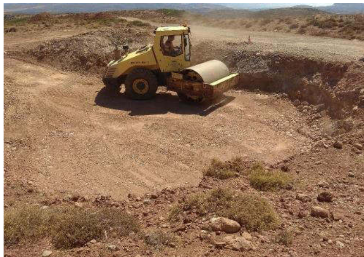
Figure 6.6- 3: Restoration of the A/G square (PPC renewable project)
