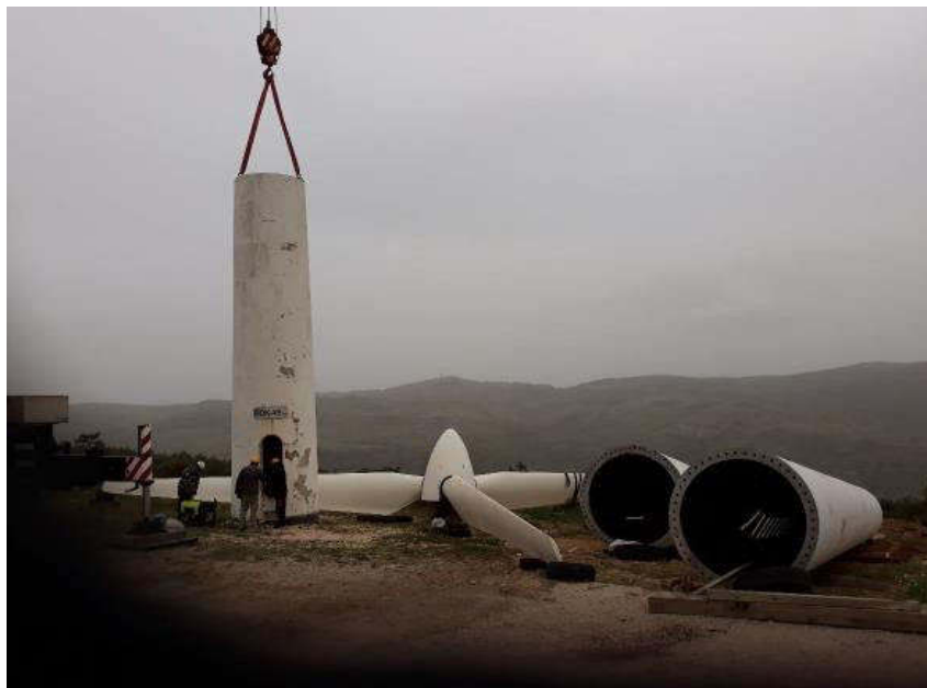
Figure 6.6- 1: Dismantling of a G/G pillar (PPC renewable project)
